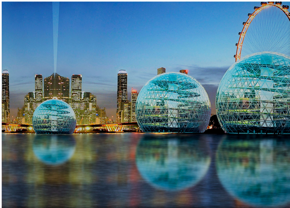
Figure 7. A proposed vertical farm by Plantagon. It comprises a helix structure placed in the center of a sphere-shape building and stretches vertically. The helix structure contains a robot belt that instead of moving thousands of plants over the whole belt, it moves each row of plants one by one. Seeds are placed in pots on the belt at the ground floor level. Then, plants are elevated to the top by an elevator and placed on the moving belt which takes them back to the ground, and by the time they reach the ground floor, plants are ready to harvest. (Drawing by author).
